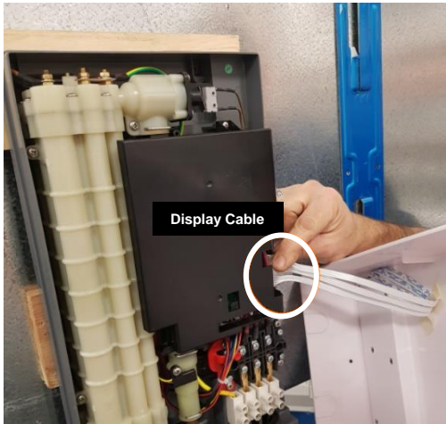
Figure 9: Removing Display Cable
